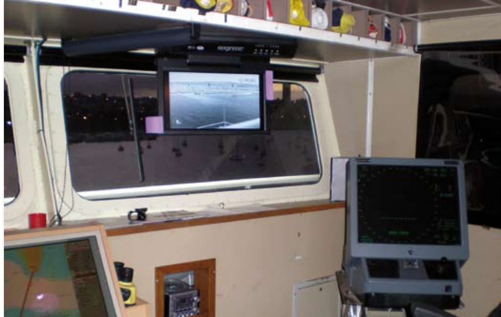
The FLIR Systems Navigator produces a crisp image which is projected on a 20" LCD screen installed on the bridge.
